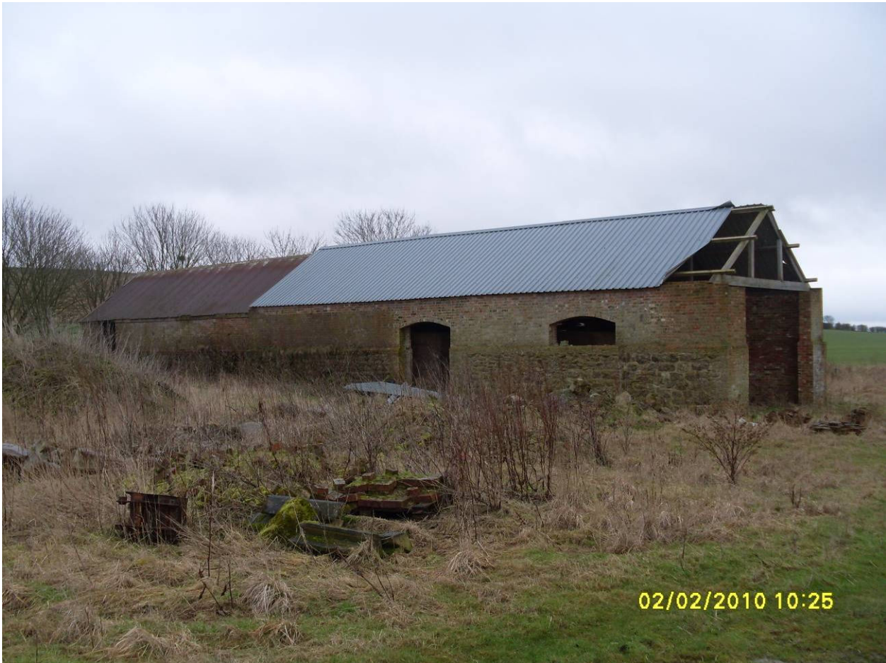
Barn 1 – as existing
